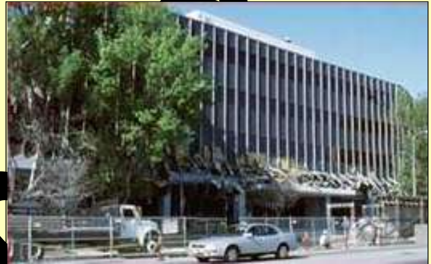
The posts could not withstand the shaking and collapsed allowing upper stories to crush second floor inhabitants.
